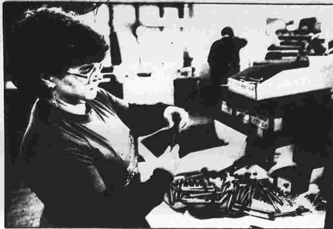
Doreen Small of 10 Camp Meeting Road places O-rings on the ends of axles.
